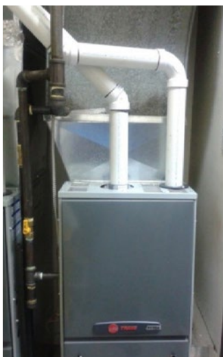
Figure 6. A newly upgraded furnace in the Region 6 office
