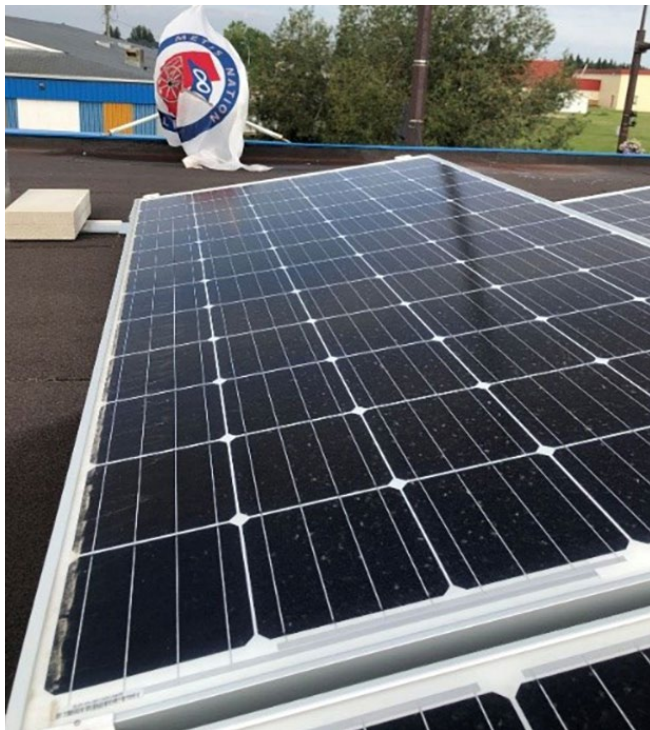
The roof top solar installation at the Region Five office in Slave Lake.
