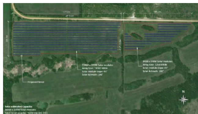
Figure 4. The Métis Crossing Solar Project in the North section of the site
