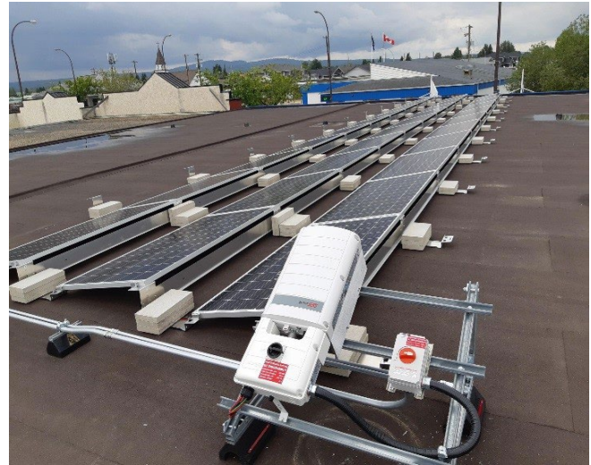
Figure 2. Region 5 office rooftop solar system
