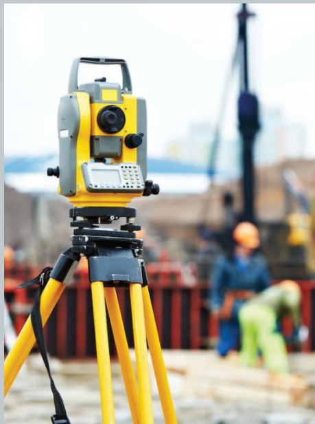
Surveying on a job sight
