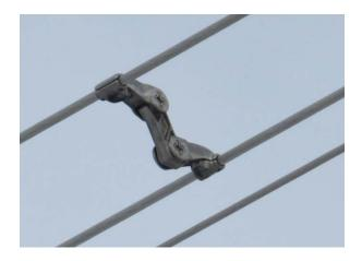
AltaLink is increasing inspections because installed spacer dampers of this type have failed on AltaLink transmission lines. Clamp bolts on the failed spacer damper did not remain secure and the clamp released from the wire, causing a portion of the spacer damper to fall to the ground. The picture below is an example of a spacer damper in a failed condition.
