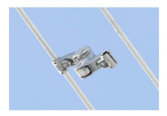
AltaLink will be inspecting spacer dampers on an ongoing basis and will address any issues as required. Inspection activities on Crown lands may include low-level helicopter flight inspections, ground level inspections and crews accessing the line from service trucks.
